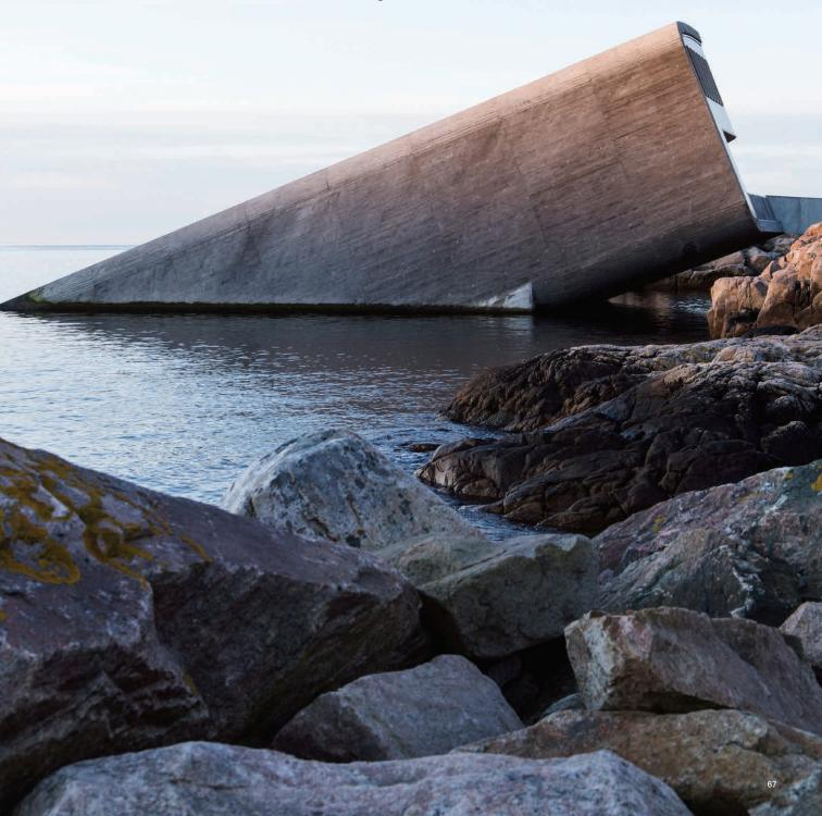
In the tiny coastal community of Båly on the southernmost tip of Norway, a 34-metre-long concrete monolith juts out of the icy waters of the North Sea. Bolted to the seabed five-and-a-half metres below, the half-sunken structure houses Under, Europe's first underwater restaurant. Guests enter by gangplank and descend an oak staircase to dine in front of a floor-to-ceiling window offering mesmerising views of frolicking seals and schools of fish.
